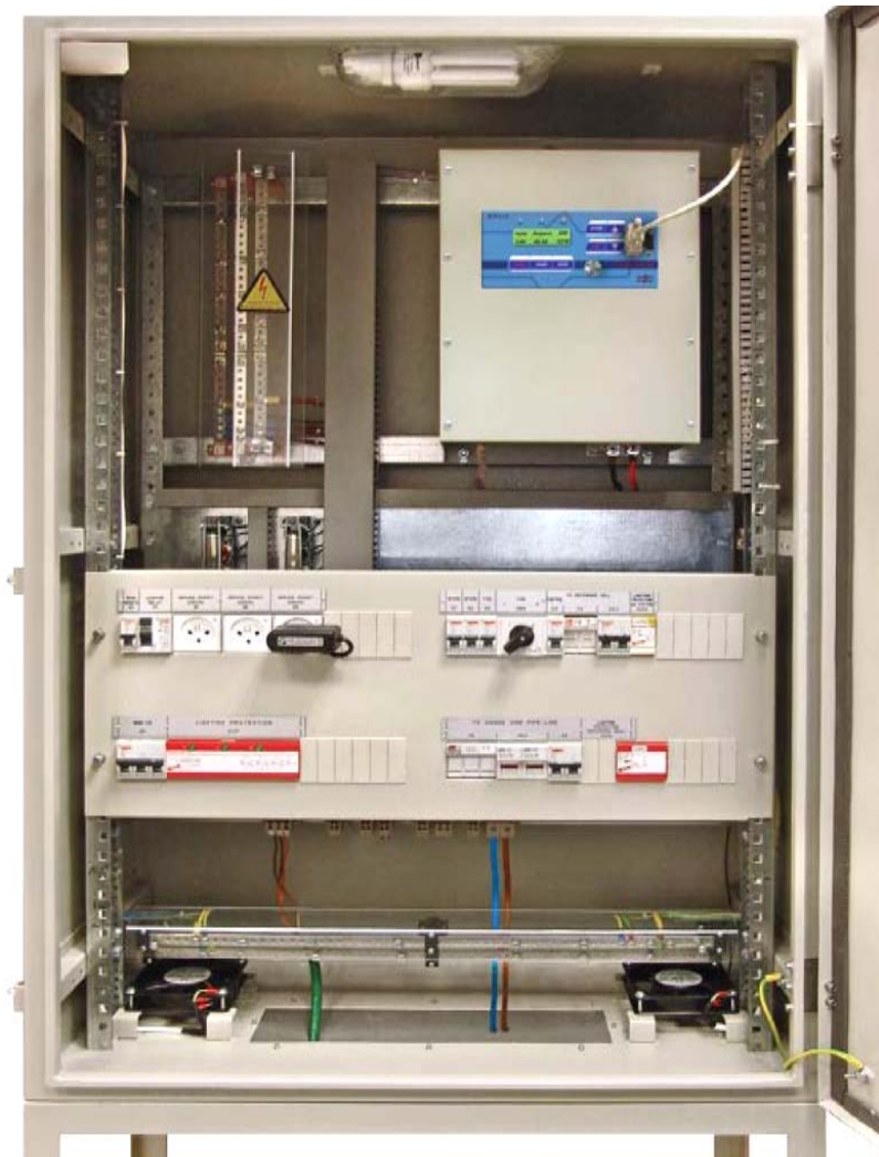
Figure 19 – An Example of an SCP-C Installation in a Cabinet
